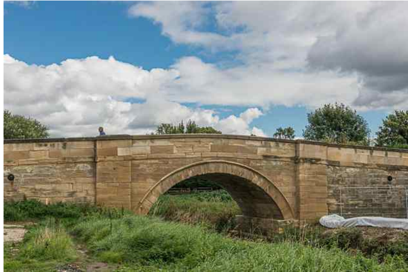
Strensall Bridge - John Carr's Bridge
